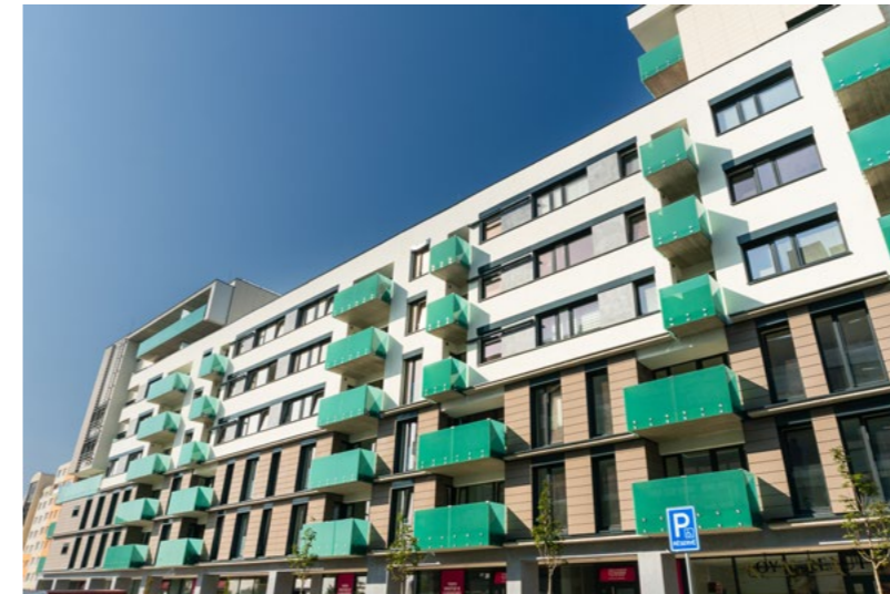
Glass railings on the housing project Smart, Prague, Czech Republic
